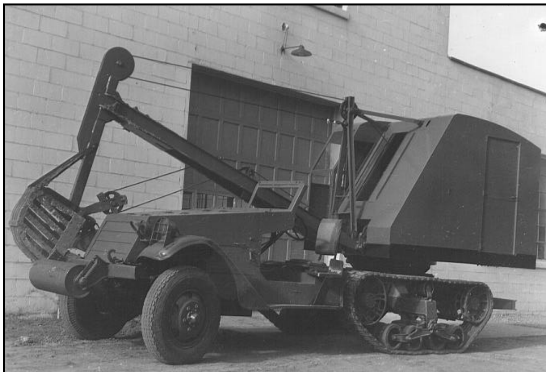
Early Bantam trench-hoe mounted on a “half-track” army surplus truck.
